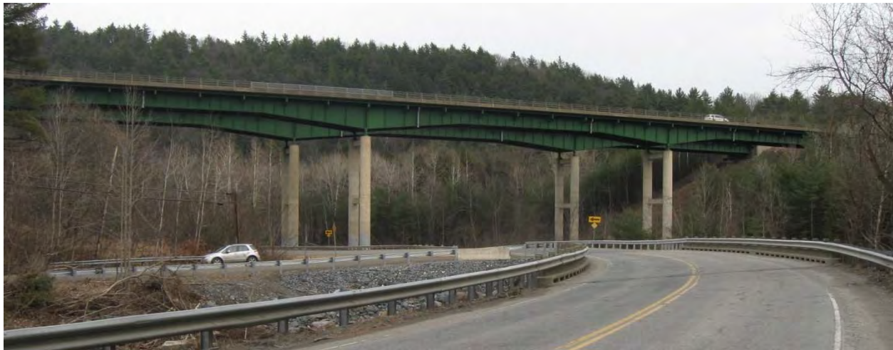
VT-44 at the “Narrows” before interstate bridge replacement in 2013 and 2014
